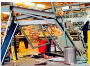
DAMAGE: A recent ram raid on an IGA Supermarket in Melbourne's West
