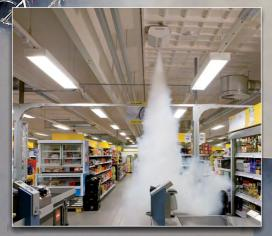
**PROTECT** Fog Cannon® is triggered: alarm and fog cannon activated.
